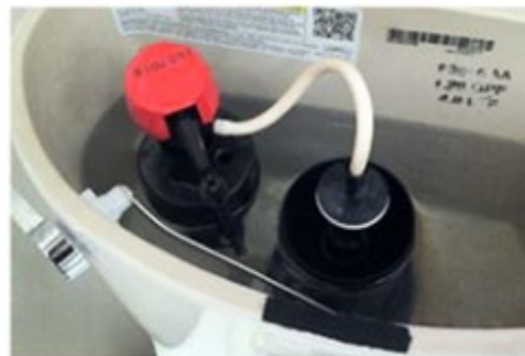
Correct (Hose Attached to Valve)
